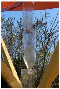
Create a tube with bottles (or other materials) to guide the harvested water (rain, dew) towards a container located in the tipi.
