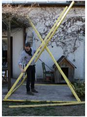
Raise 2 pieces of wood 4000 mm (from step 2) Screw (or assembly) them on the other pieces of wood (from step 4)
